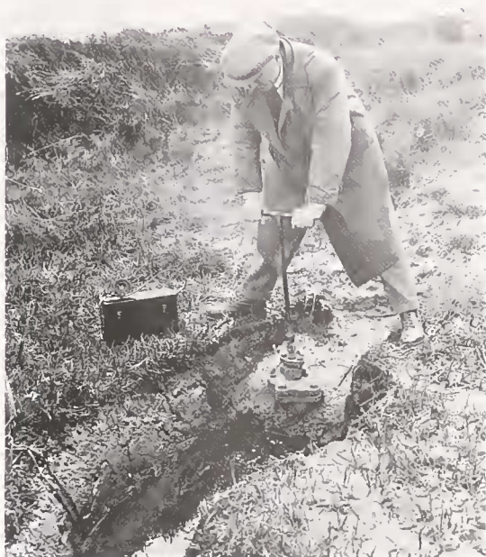
Fig. 20 Draining a salt-marsh area by opening a sluice valve during low tide
